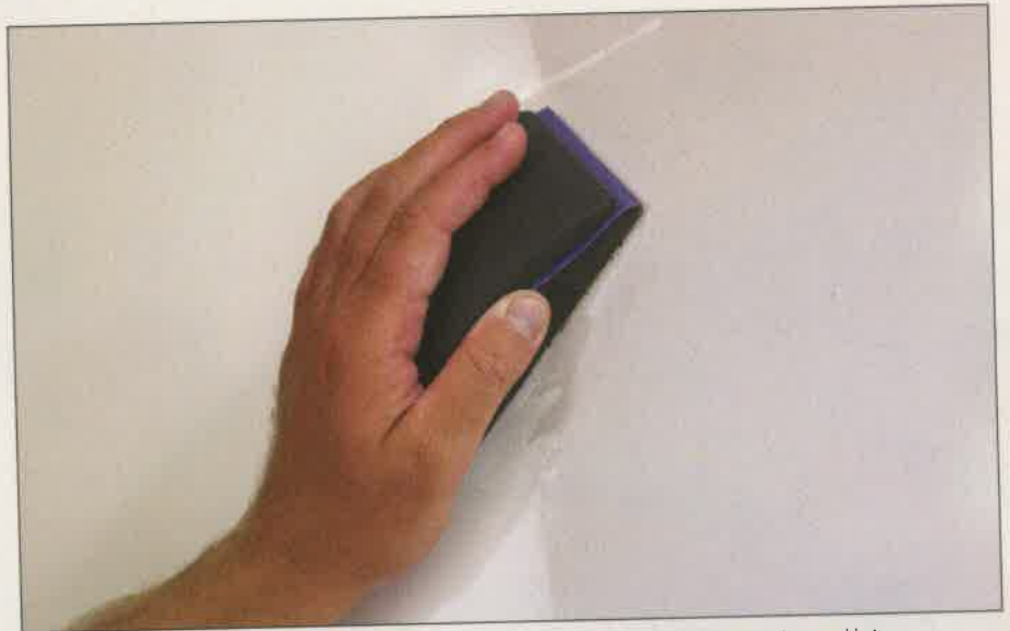
Rigidity is the key to skiving off bumps and imperfections. A rubber sanding block fitted with sandpaper is a good bet.
