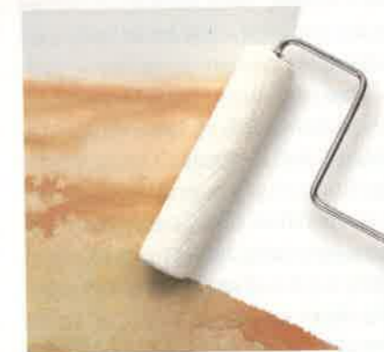
● Blocking water stains.
